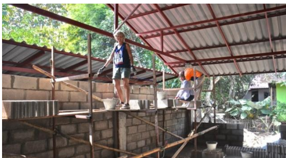
Members of the building team hard at work.
